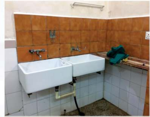
Prep Room Before
